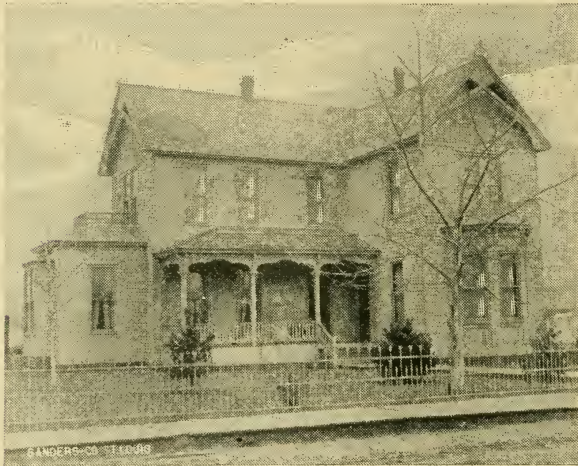
RESIDENCE OF R. H. JONES.
