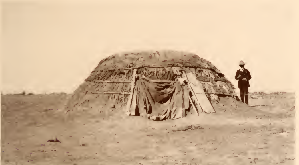
Plote 5. Completed house covered with brush and earth. Convos in the doorway is a modern touch.
