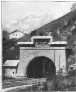
Abbild. 51. Arlbergtunnel (Ostmund).
