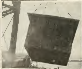
Placing Hatch Trunks in position, for salvaging s.s. Canadian Recruit .
