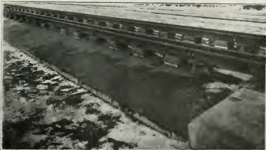
Fig. 1. 200-Ton Track Scale, C.P.R. General View, Waterproof, Tapered Scale Deck.
