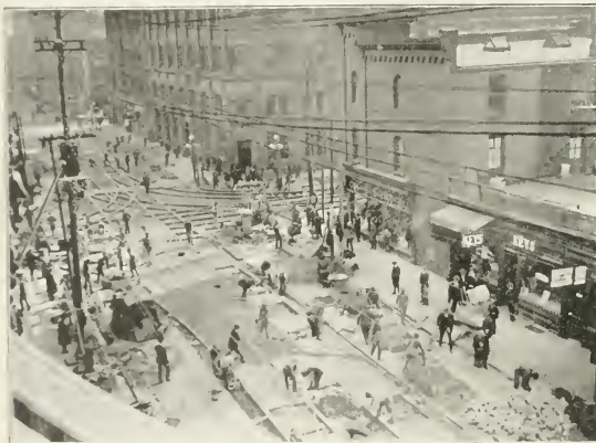
Toronto Transportation Commission's Track Reconstruction, Queen and Victoria Sts., looking south.
