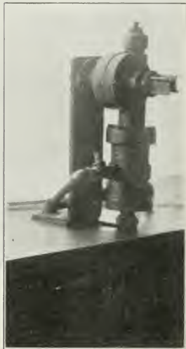
Grinding in triple valve emergency check valves: valve in position for grinding.
