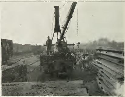
Fig. 2. Air Operated Rail Handling Machine.
