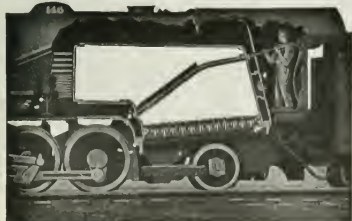
Lagonda Cleaner Removing Scale from Arch Tubes.
