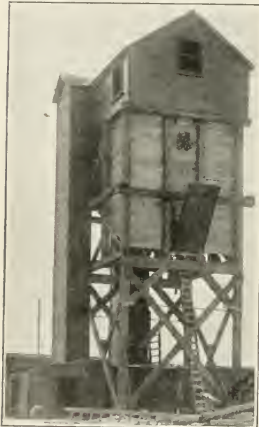
Fifty-ton, Single Track, Gasoline Drive, Coal Handling Plant, Canadian Pacific Railway, Guelph, Ont.
