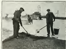
Below: Pouring final coat of hot Barrett Specification Pitch and embedding thick wearing surface of gravel or slag after entire roof has received four plies of felt and pitch.
