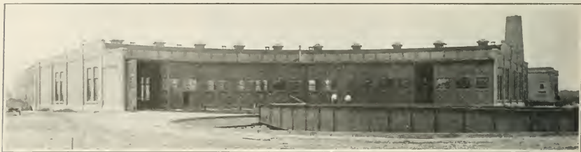
Locomotive House, Leaside Shops, Canadian National Railways.
