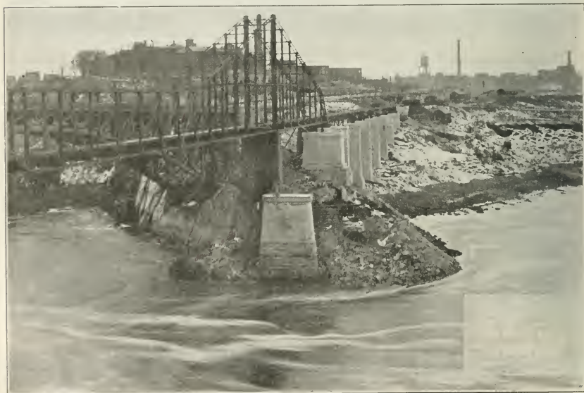
C.P.R. Cantilever Bridge, St. John, N.B. General view, looking west, Dec. 31, 1920. This illustration shows the western main pier of the new cantilever bridge, the west anchor pier, and the piers for the western approach viaduct, then a portion of the present C.P.R. cantilever bridge and a portion of the New Brunswick Government's bridge for vehicular, pedestrian and electric railway traffic. On the main pier in the foreground will be seen the granite facing, between high and low water marks.
