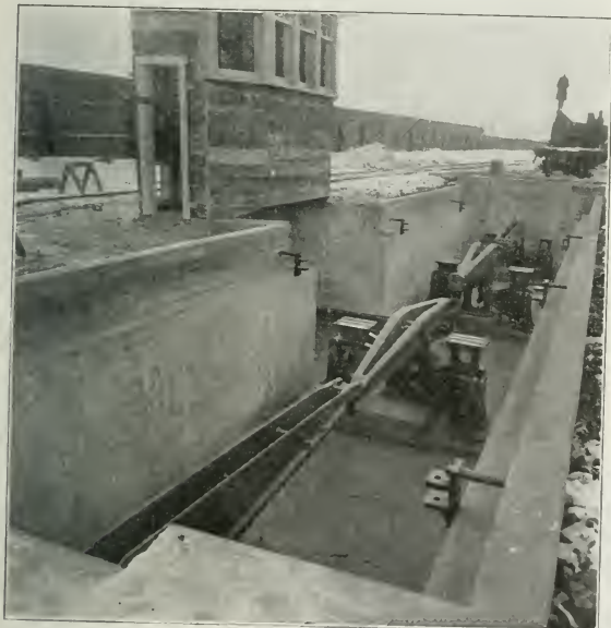
Fig. 2. 200-Ton Track Scale, C.P.R. General View of Pit, showing Scale. See pp. 289 and 290.
