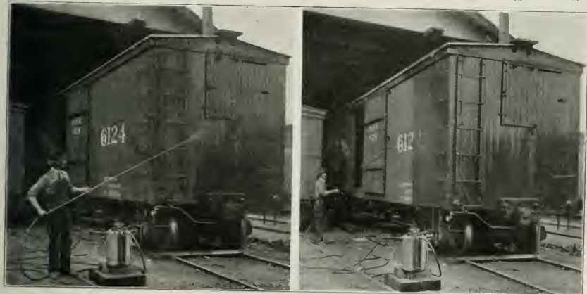
British Columbia Electric Ry. Car Painting Methods.
