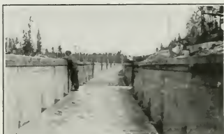
Improved Car Unloaded by Top Plow. Has no Ballast to be Shovelled out by Hand.
