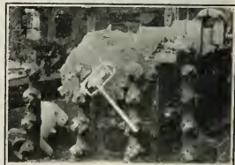
Changing Superheater Joints.
