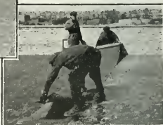
Below: Pouring final coat of hot Barrett Specification Pitch and embedding thick wearing surface of gravel or slag after entire roof has received four plies of felt and pitch.
