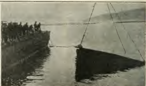
Placing Hatch Trunks in position, for salvaging s.s. Canadian Recruit .
