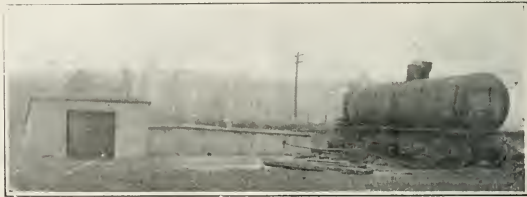
Fig. 1. Oil Storage House, Canadian National Rys. Leaside Shops, Toronto.
