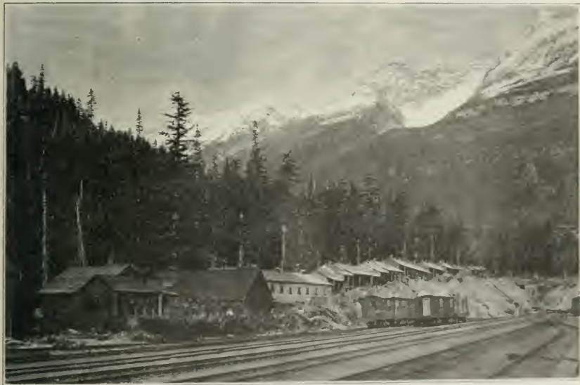
Portion of Construction Camp, for Concrete Lining of Connaught Tunnel, C.P.R.
